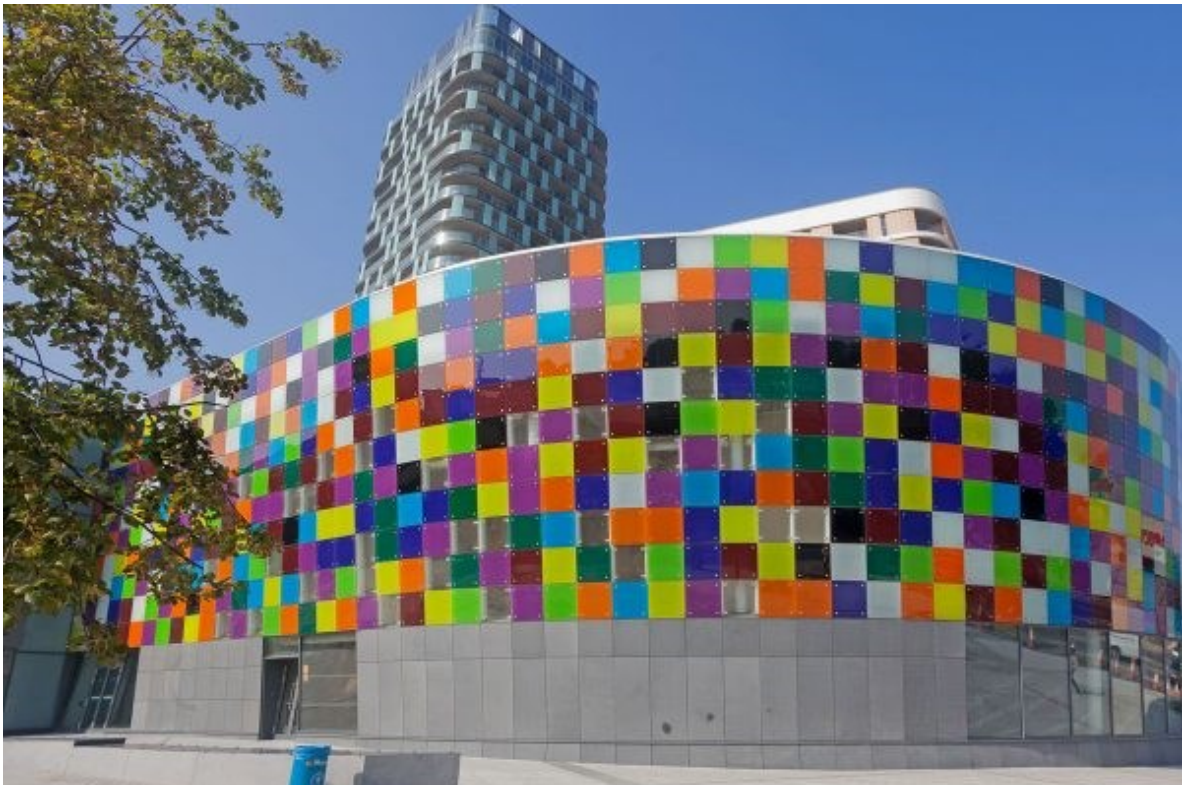
Lewisham Recreation Centre
