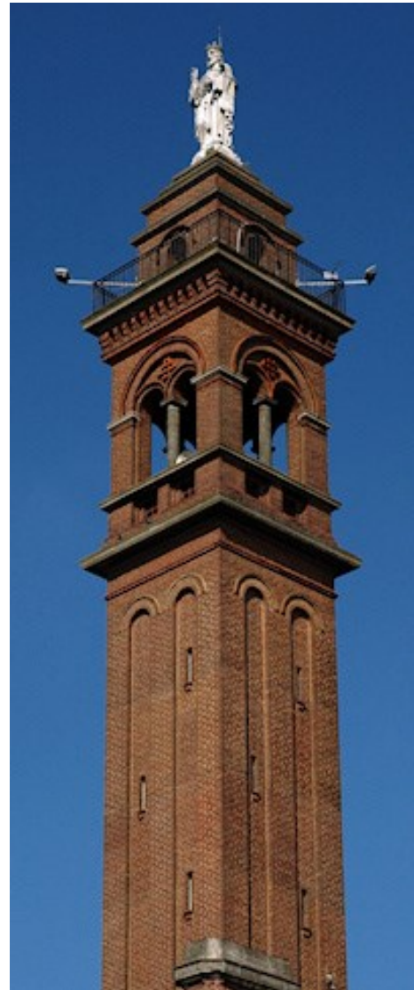
St Saviour's Church Tower
