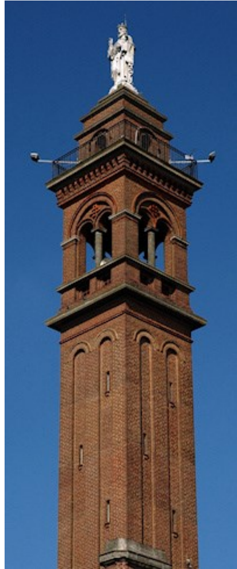
St Saviour's Church Tower
