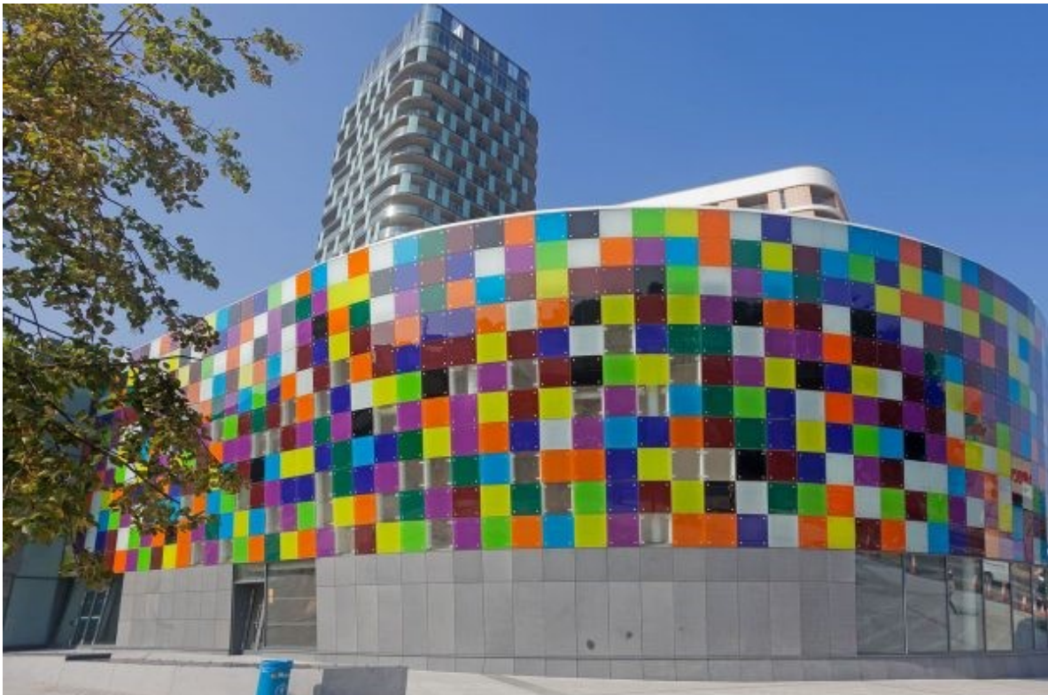
Lewisham Recreation Centre
