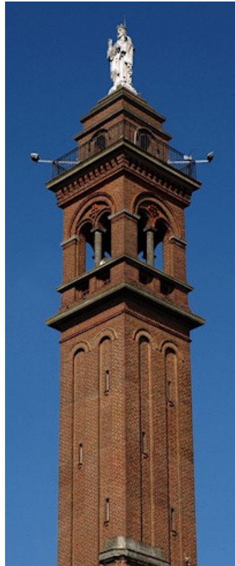
St Saviour's Church Tower
